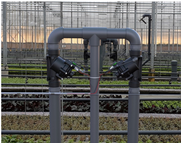
[1] The BERMAD Model IR-11T-N5-2W opens and closes drip-tight in response to an electric signal, which causes the solenoid to open or close the valve's internal hydraulic loop.
